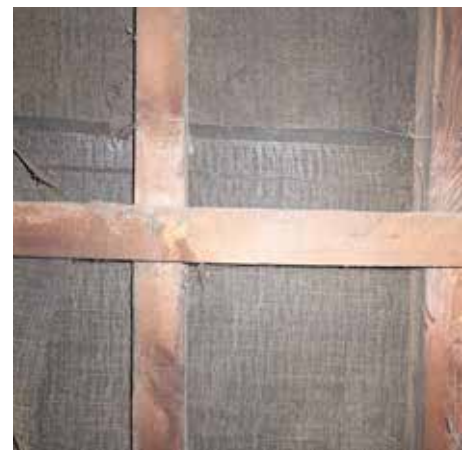
(xii) New roof timber/ felt
